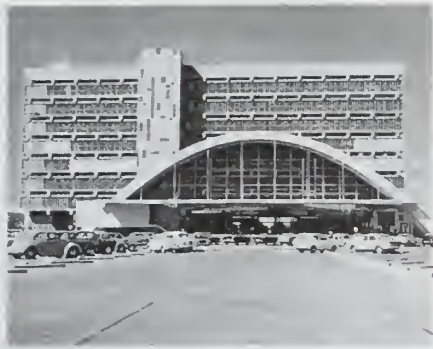
The railway station, Beira, Mozambique
